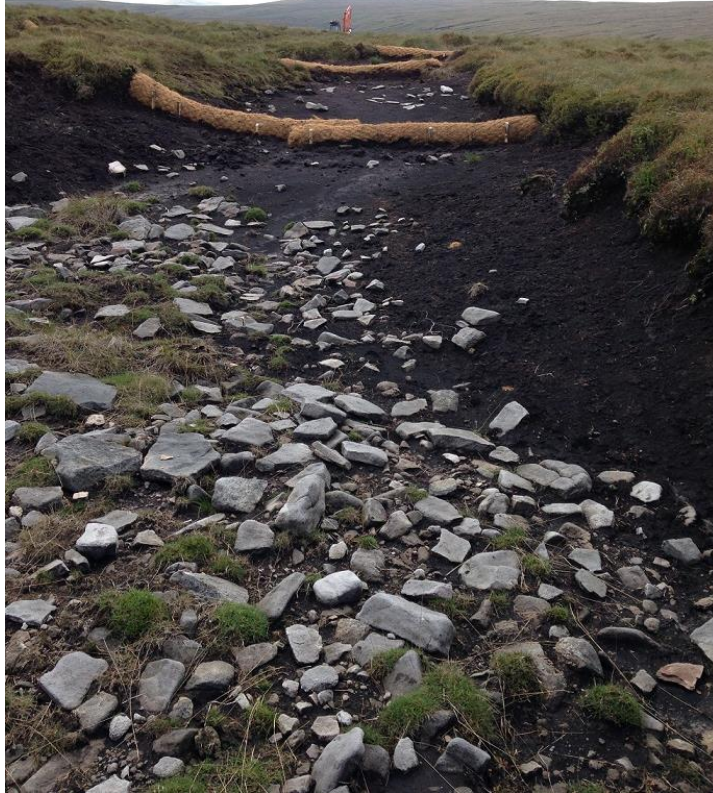
Coir logs across low wide gully
