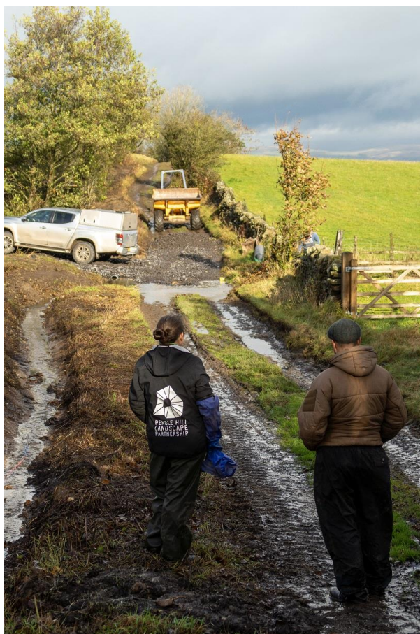
Checking on the repairs to Coalpit lane
