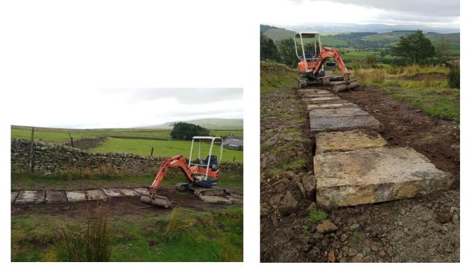
The new flag path being installed at the foot of Pendle, aiming to create a more resilient path for walkers
