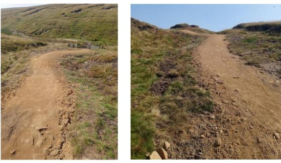
The track after resilience work, showing the repaired surface and profile
