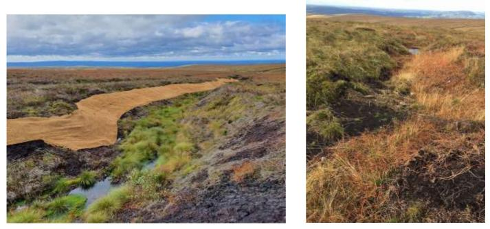
Geo-textile laid to protect the gully side, ready for seeding & brash; revegetation on site 2 years after the original work
