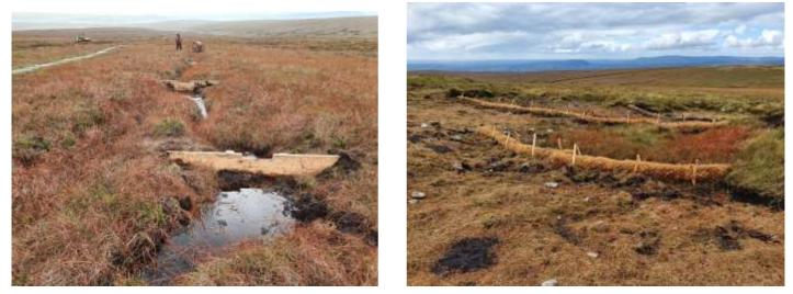
New timber dams installed in the narrow gullies and new coir logs in place on the summit: both will slow the flow
