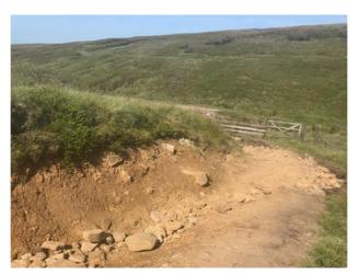
The track to Ogden Clough before repairs - showing the deep washout area
