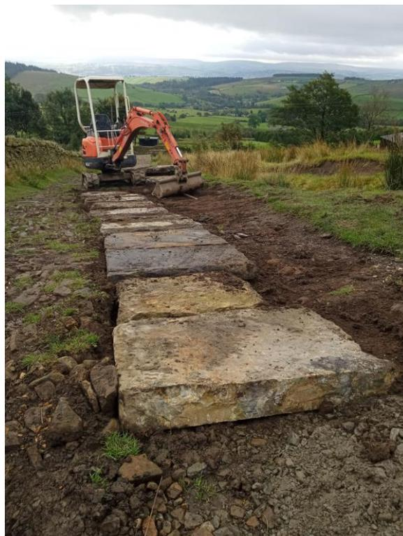
The new flag path being installed at the foot of Pendle, aiming to create a more resilient path for walkers
